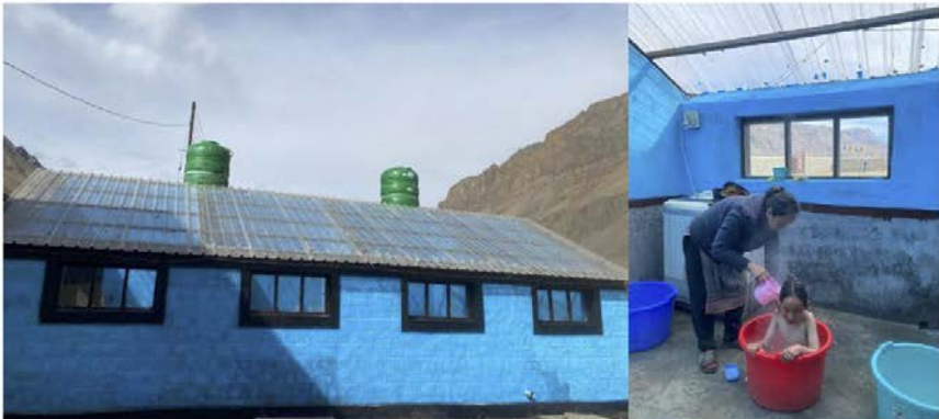
Translucent panelling on the roof at Rewa Primary School keeps the inside warm when the outside is freezing
